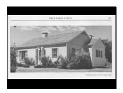
In some parts of the country, American Small Houses were built using experimental construction materials and techniques. This house was built using plywood for the exterior sheathing ...
