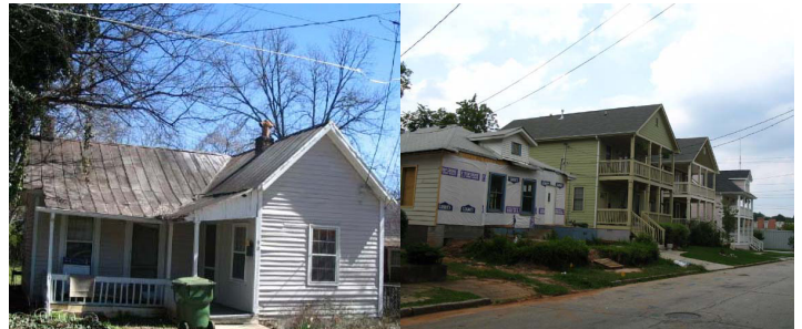
The gabled ell cottage on the left maintains its historic integrity while new construction on the opposite side of Chester Avenue no longer conveys the historic landscape of the community.
