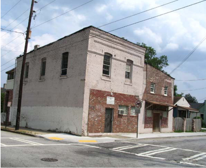
This commercial building in the Reynoldstown Historic District is adaptively used as the Reynoldstown Baptist Church today. Photo by Jeanne Cyriaque
