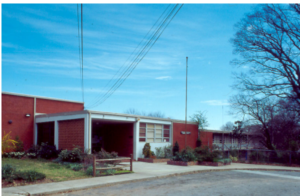
The former Reynolds Elementary School was designed in the International Style. This type of one-story school construction was defined by simple geometric forms and lack of ornamentation.
