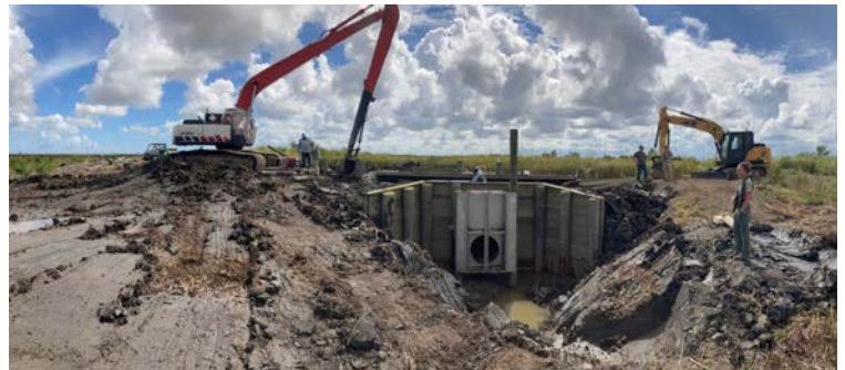
Rhett's Island waterfowl impoundment repairs.
