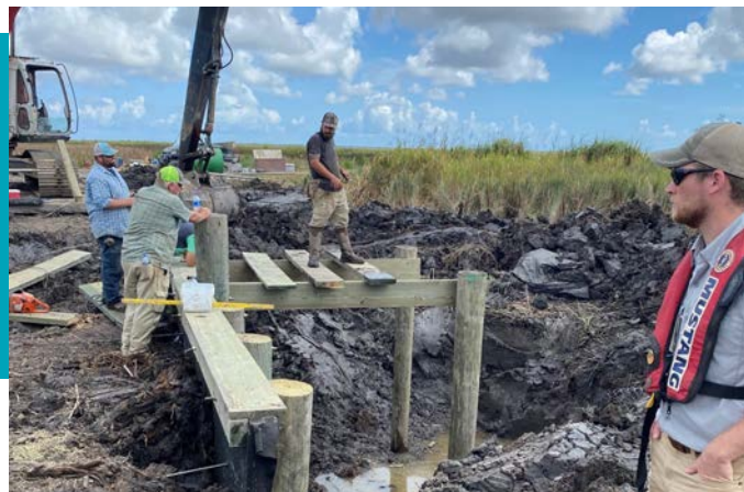
Ongoing repairs to infrastructure at Altamaha WMA.
