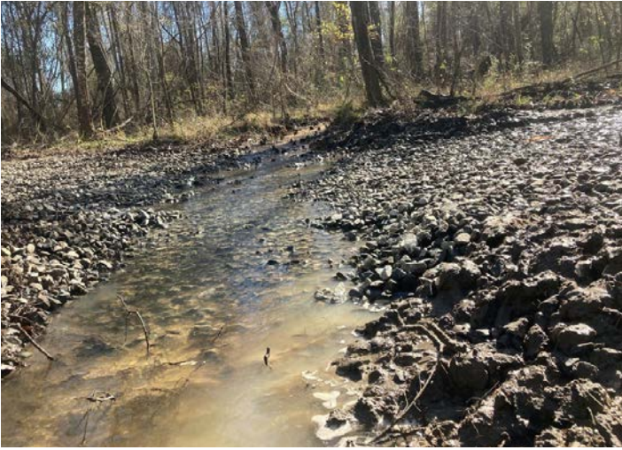
Low water crossing installed at Bullard Creek WMA.
